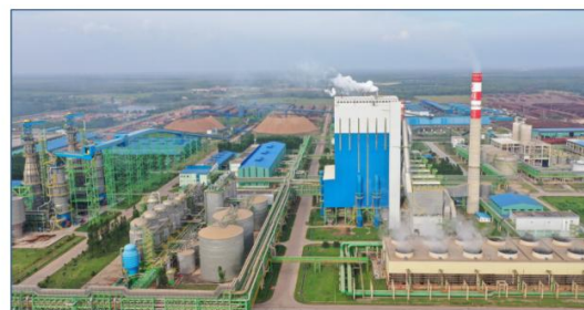
Pulp Production Facility
