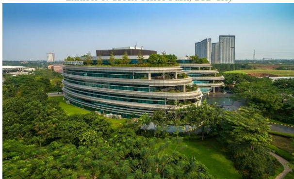
Exhibit 6. Green Office Park, BSD City
